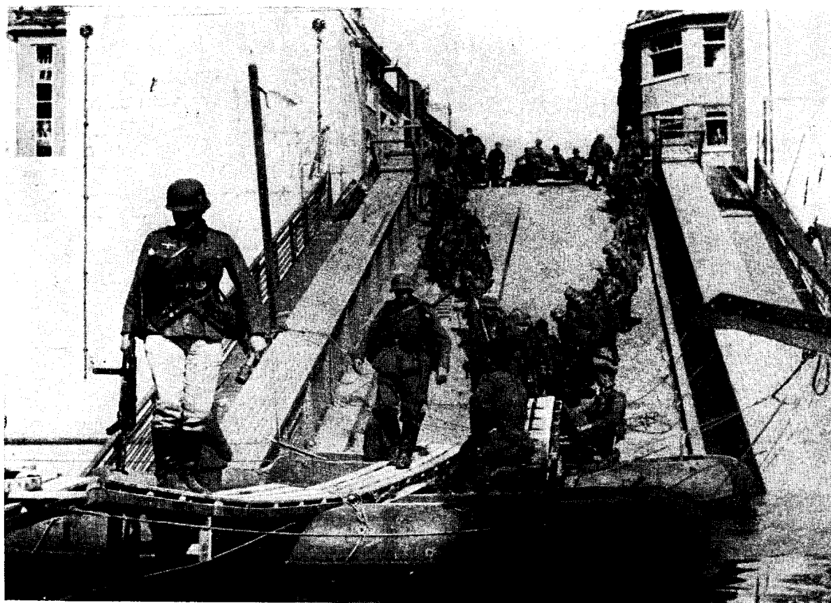
Figure 96.—Track bridge and medium pneumatic boat.
