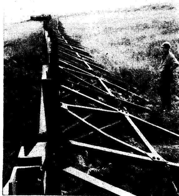
Figure 17.--German Element "C" joined to form antitank obstacles.
