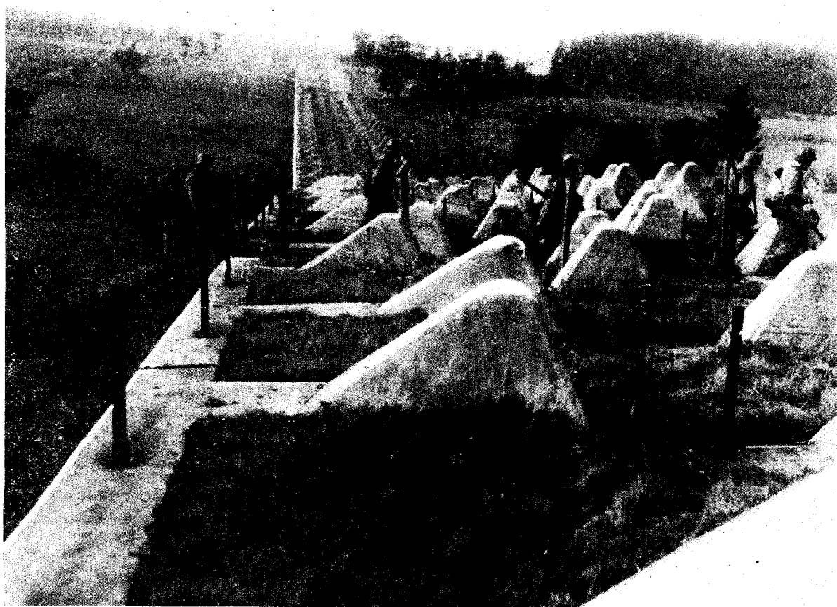
Figure 16.--Dragon's teeth showing concrete foundations.
